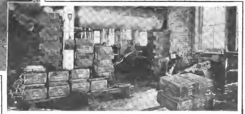
The furnace room of the Holley plant. Six oil furnaces melt the metal in crucibles from which it is carried in ladles to the molds
